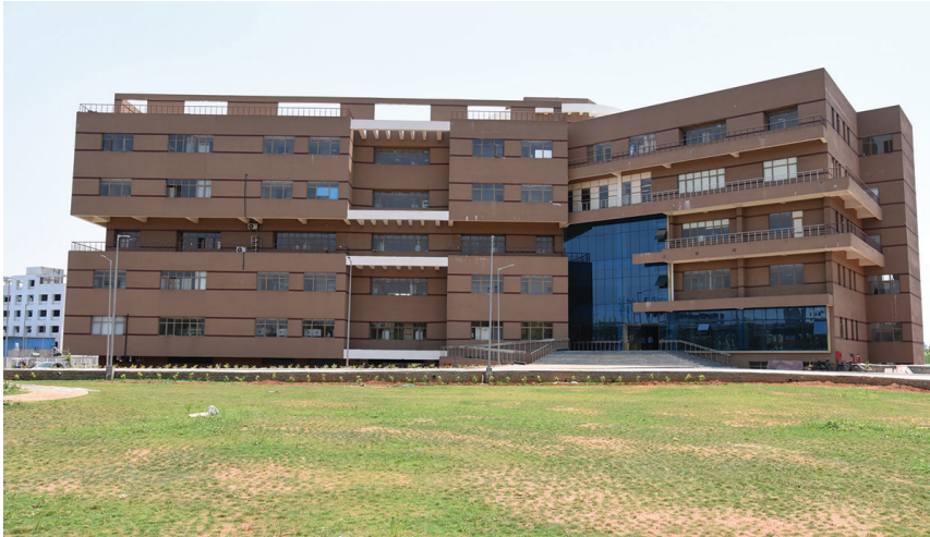
CDFD Lab Building in Uppal Campus
